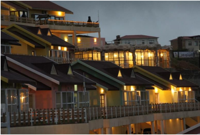
General Construction (Permanent Concrete and Prefab) .
